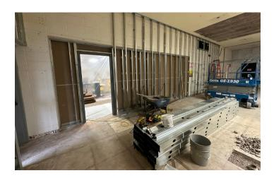
One exciting piece of the project for staff has been the removal of the moveable wall between the meeting room and staff offices. The moveable wall has been replaced with a permanent wall, adding extra wall space and more outlets on the staff side.
